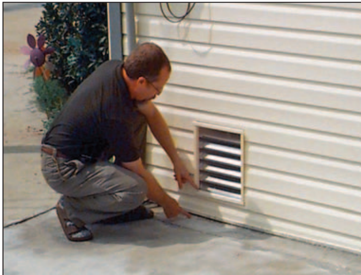
Figure 6-43. Example of flood vents
