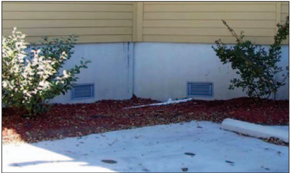
Figure 6-42. Example of flood vents
